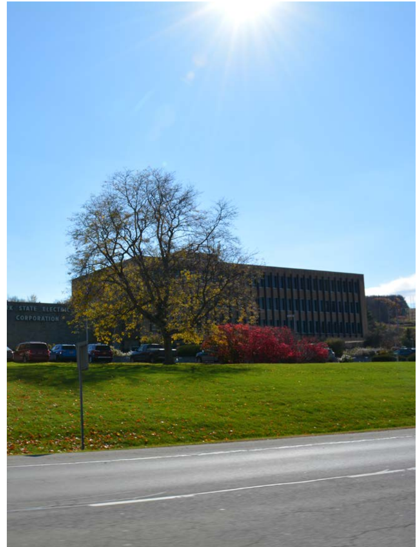
PHOTO: NYSEG BUILDING NYS Route 13
